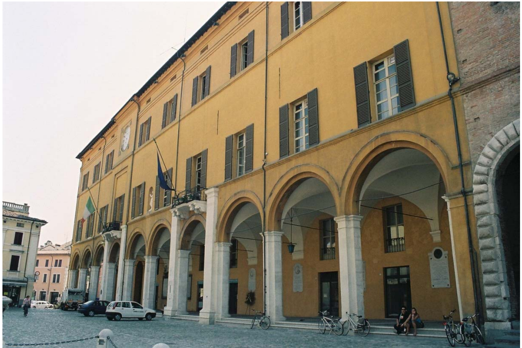
Figure 71. North front. Palace, Cesena.
