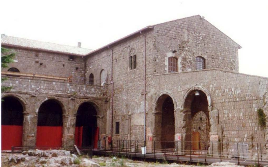
Figure 44. Fortified palace. Montefiascone. Courtyard.
