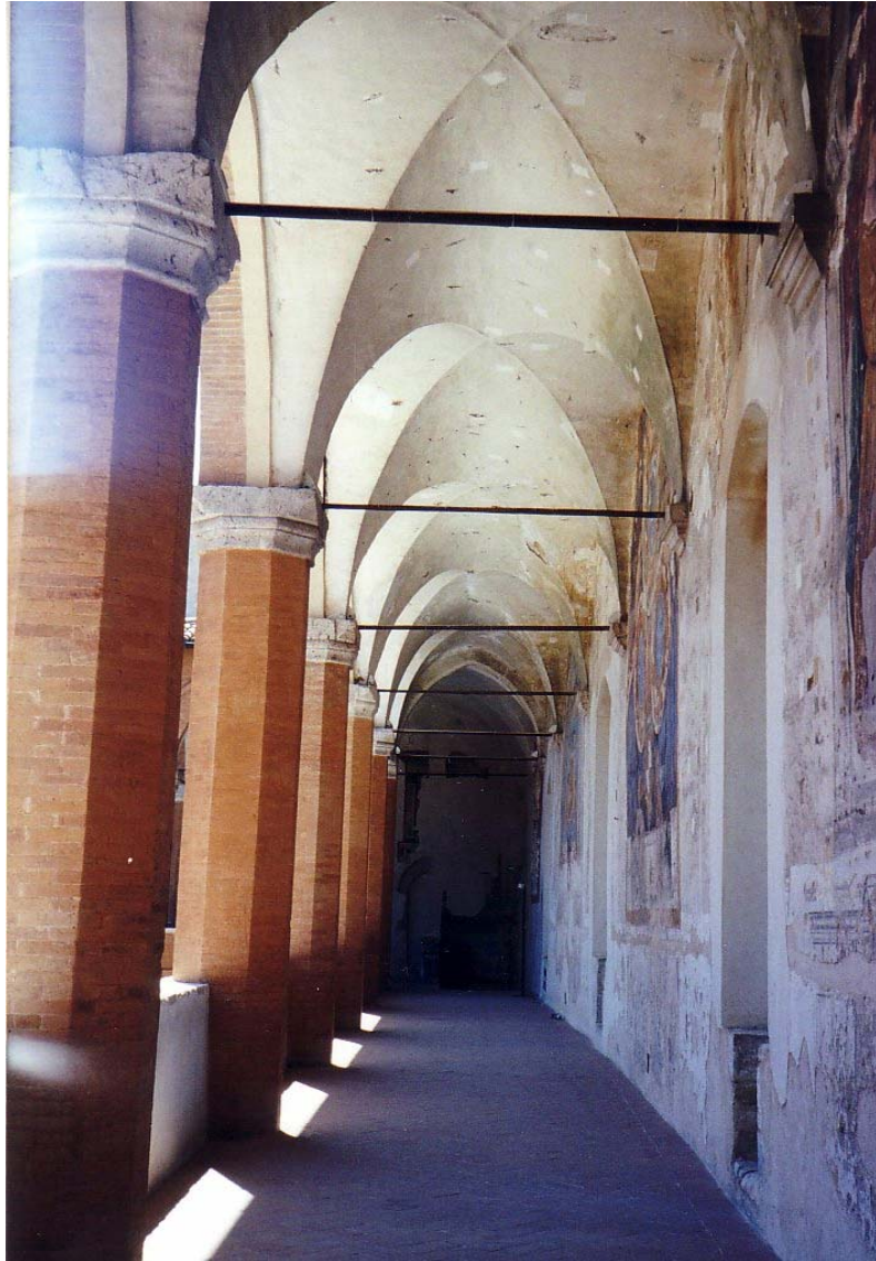
Figure 60. Upper loggia. Residential courtyard. Rocca, Spoleto.
