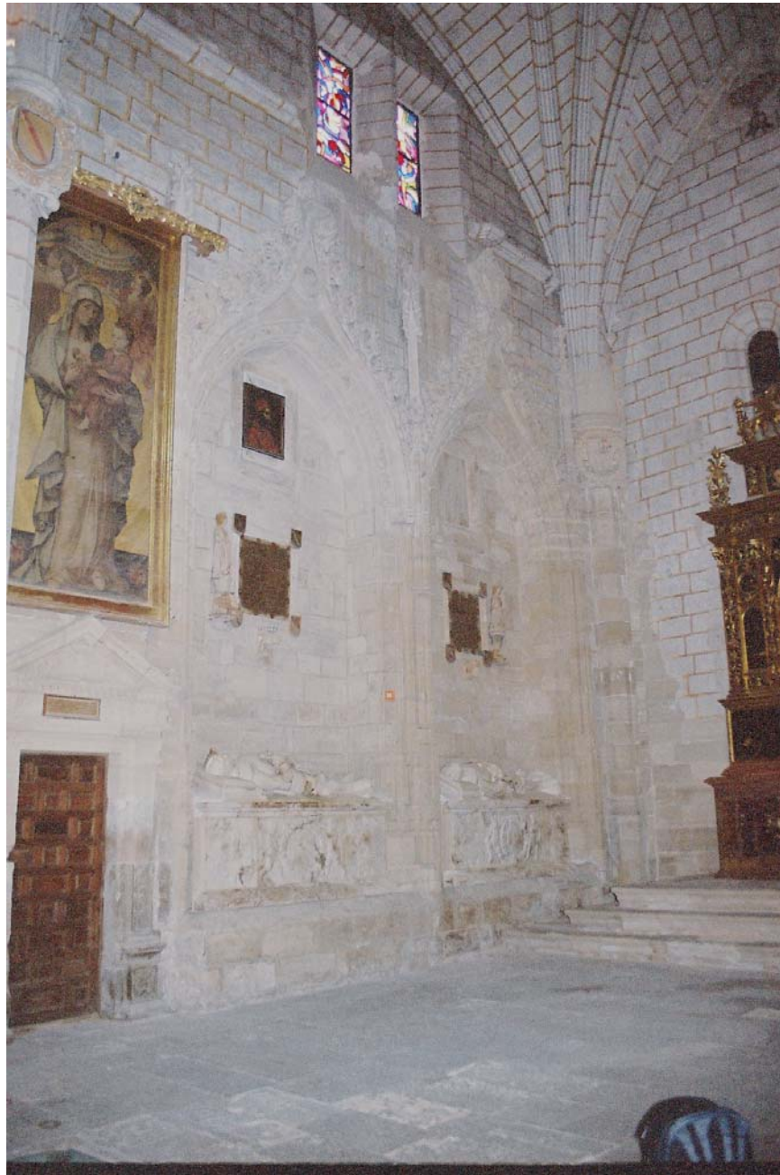
Figure 5. Cuenca cathedral. Interior. Albornoz family chapel. View from the south entrance.
