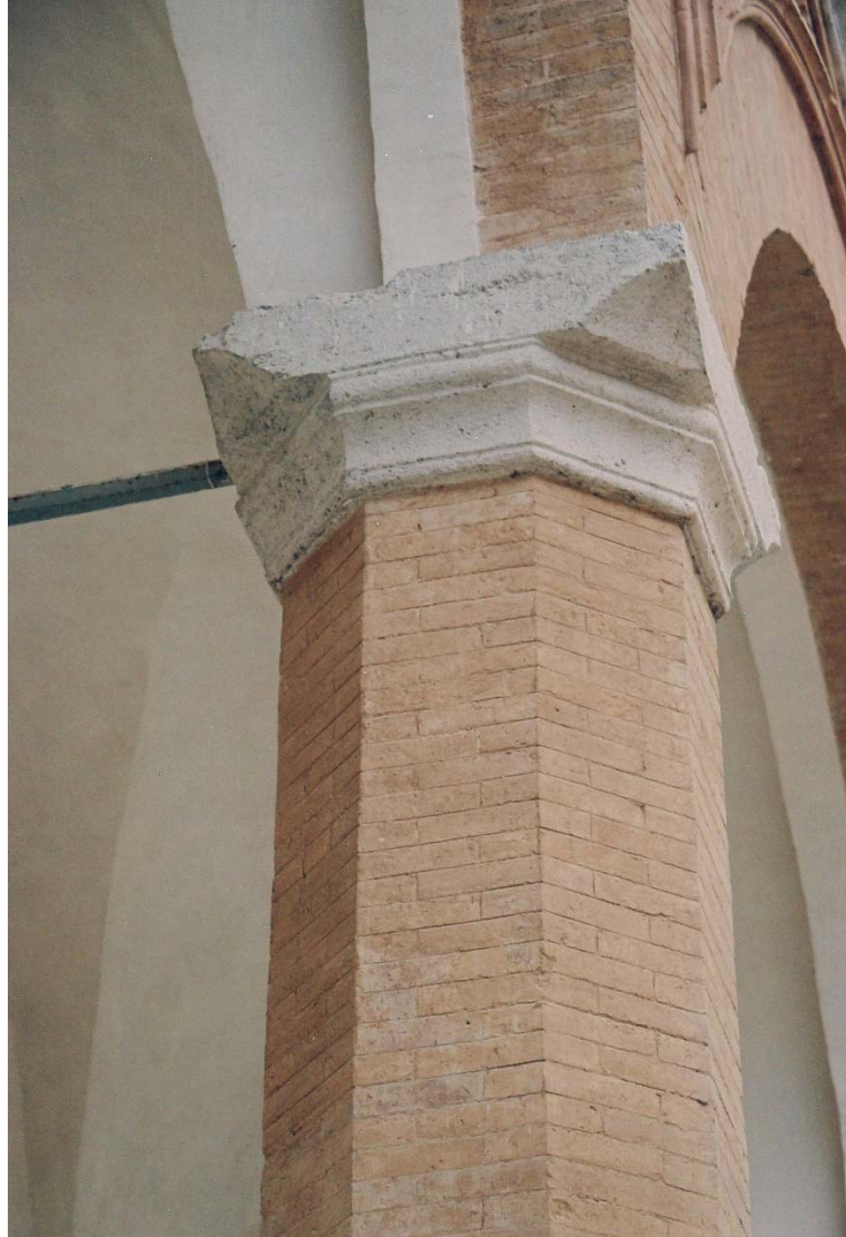
Figure 59. Pillar in residential courtyard. Rocca, Spoleto.
