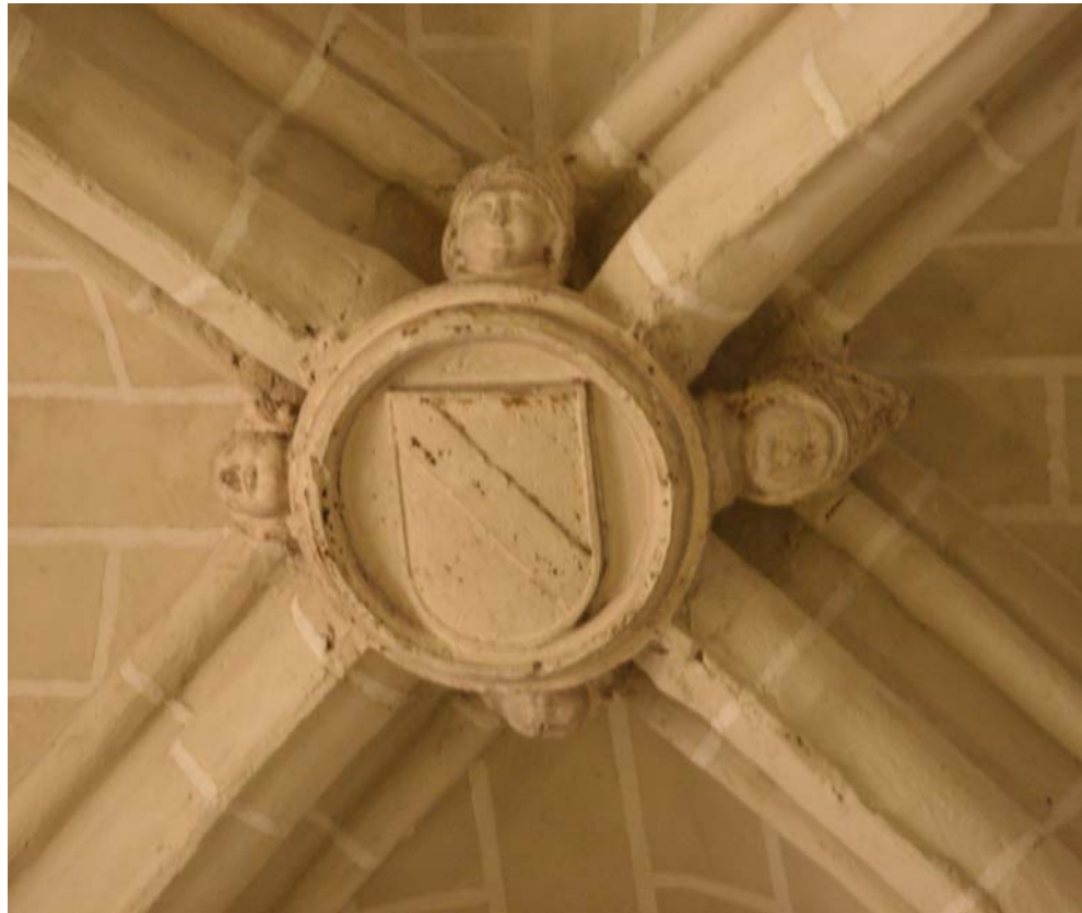
Figure 24. Toledo Cathedral. Interior. Key stone on vault of north aisle, decorated with Albornoz heraldry, 1338-1350 [Tom Nickson]
