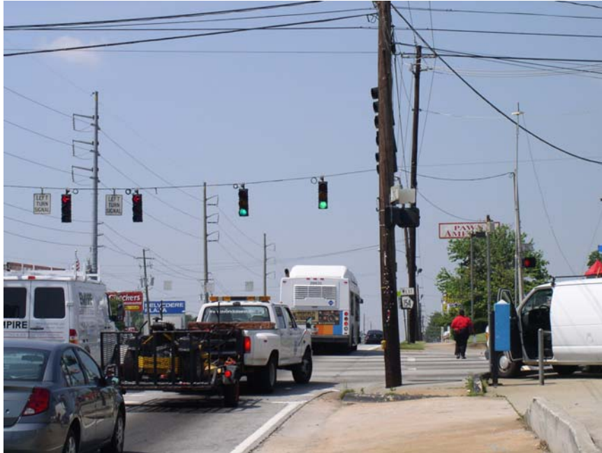
Figure 94: Roadside antenna at the intersection of Memorial Drive and Candler Road.
