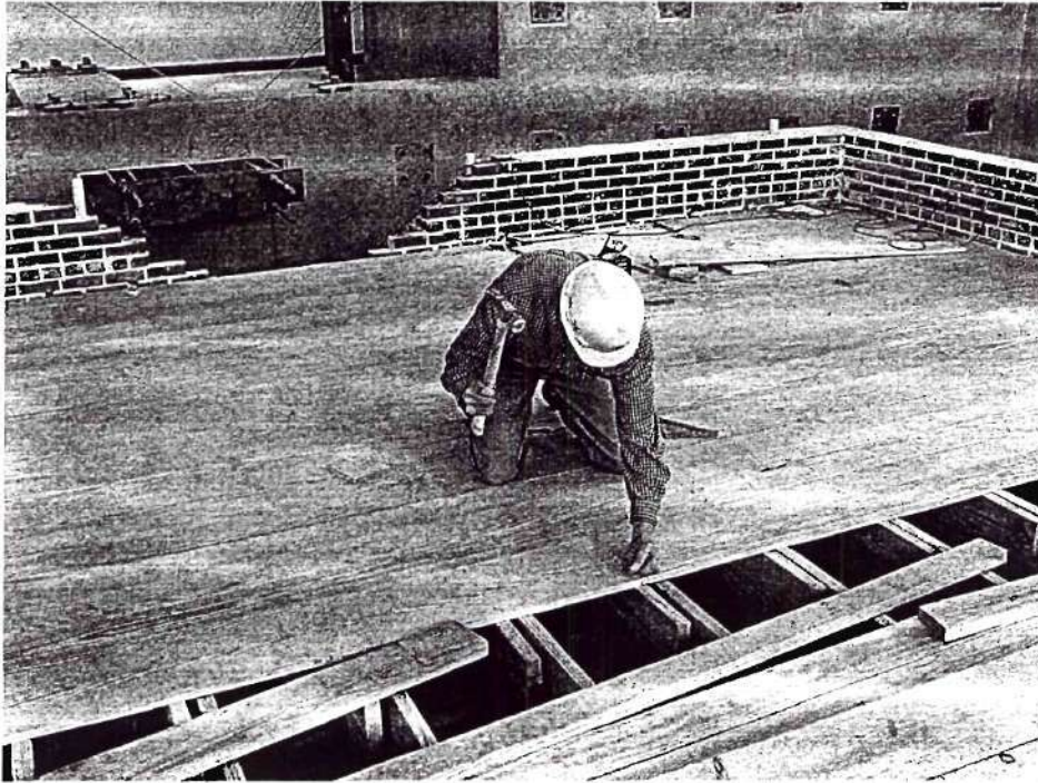
Figure 3.24. Construction of the floor and roof diaphragms.
