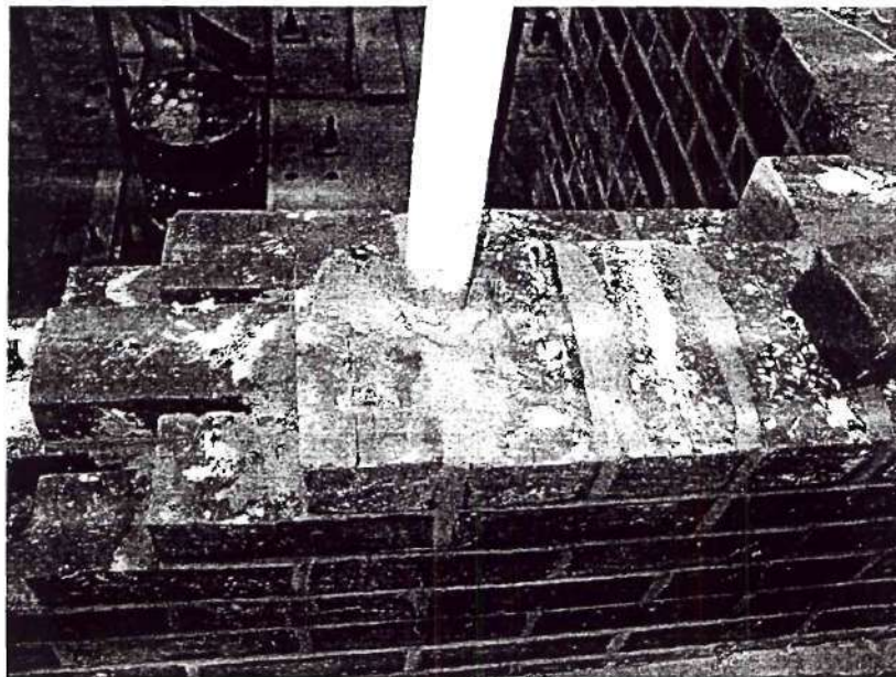
Figure 3.19. PVC tubes used to leave the holes in the wall
