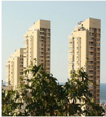
Figure 6.1: Perspective view of the three towers W, V and X of the Cap-sur-ville project in Beirut (Lebanon).
