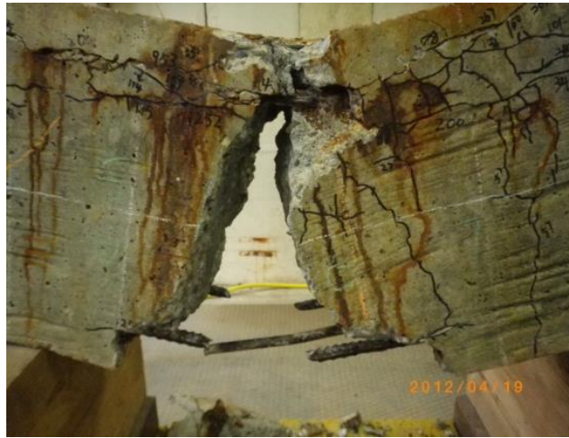
(a) Failure of corroded beam B2C13-1 (The middle bar is designed to be the handle)
