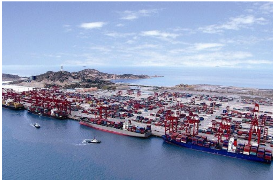
Figure 1.2: Layout of the Container Terminal YANGSHAN, Shanghai, China. http://www.dianping.com/photos/7635647
