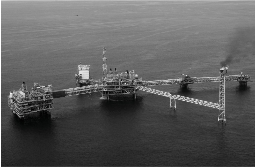
Figure 1.4: Aerial view of the Total offshore platform located in Amenem (Niger's Delta). The natural gas obtained as a byproduct of the oil extraction is burnt (right side of the picture). (Pius Utomi Ekpei/AFP/Getty Images, www.theatlantic.com )
