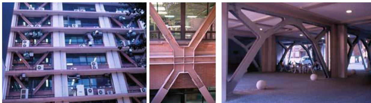
Figure 1-20: Exemple de contreventement métallique (University of Tokyo buildings) (Fardis 2009)
