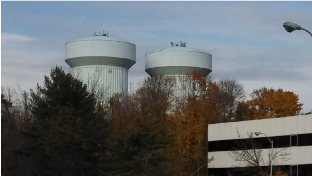
Picture 1: Mount Pleasant Water Tower
