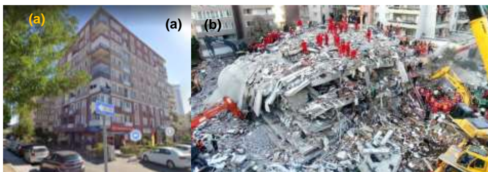
Figure 85: Riza Bey Apartments: (a) before (Google Maps) and (b) after the earthquake ( https://www.haberler.com/riza-bey-apartmani-nerede-riza-bey-apartmani-13705665-haberi/ )
