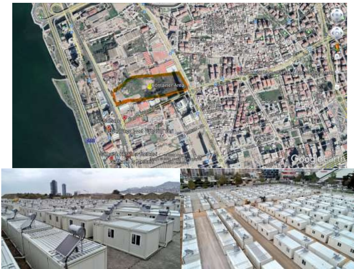
Figure 117: Temporary housing (photographs from https://twitter.com/AFADBaskanlik/status/1329360425616617472 )
