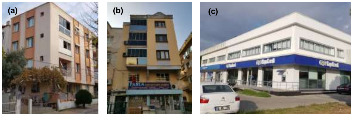
Figure 80: Good response of (a) – (b) RC frames with infill masonry walls and (c) RC precast industrial building
