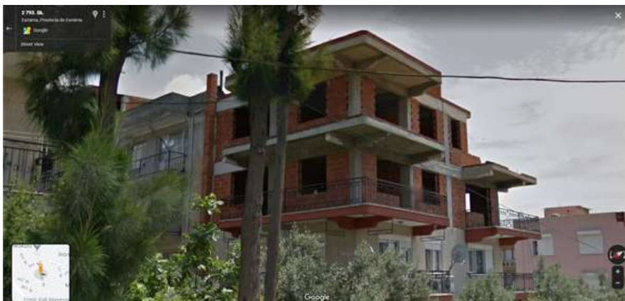
Figure 76: Street view from Izmir – reinforced concrete first and second extension under construction
