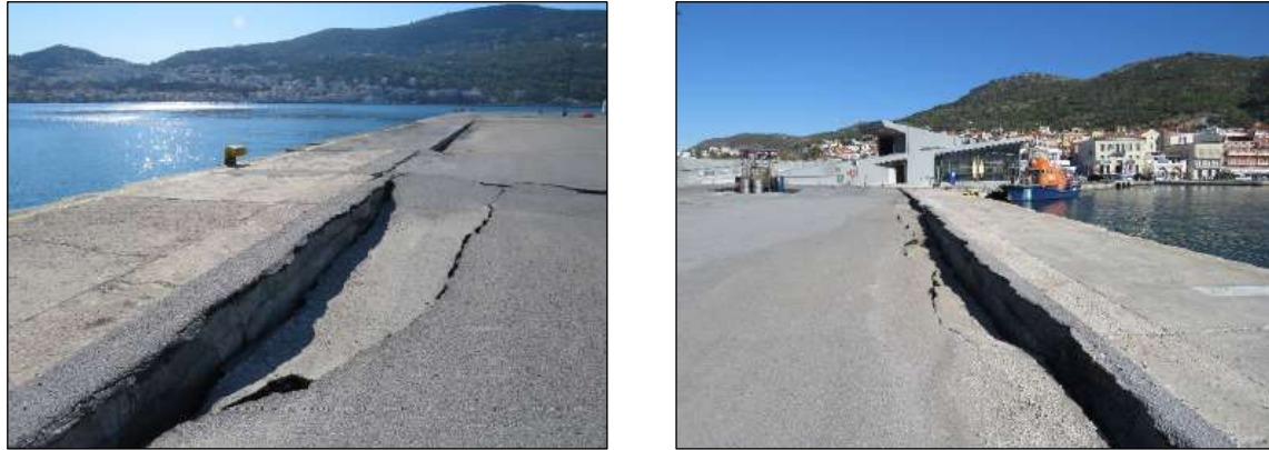
Figure 44: Significant damage was observed on Vathy ports of Samos (Lekkas et al., 2020)
