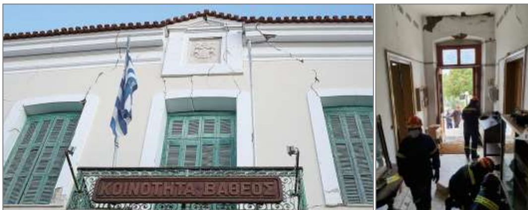
Figure 73: Severely damaged historical building of the town hall of Vathy (photo credit: Facebook page - Kathimerini)
