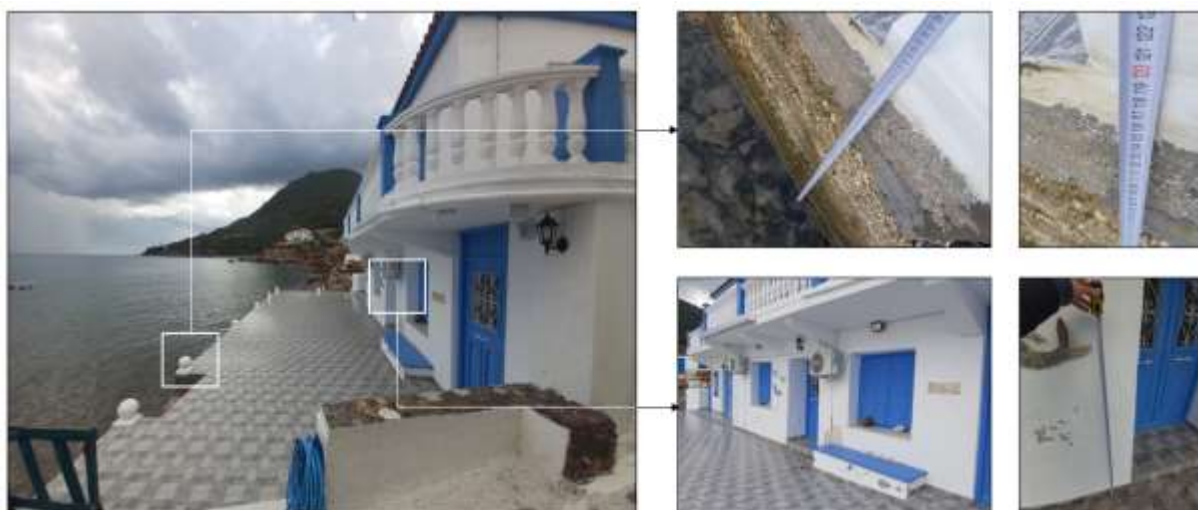
Figure 99: House at Ayios Nikolaos beach: measurements by EEFIT Greek field crew.
