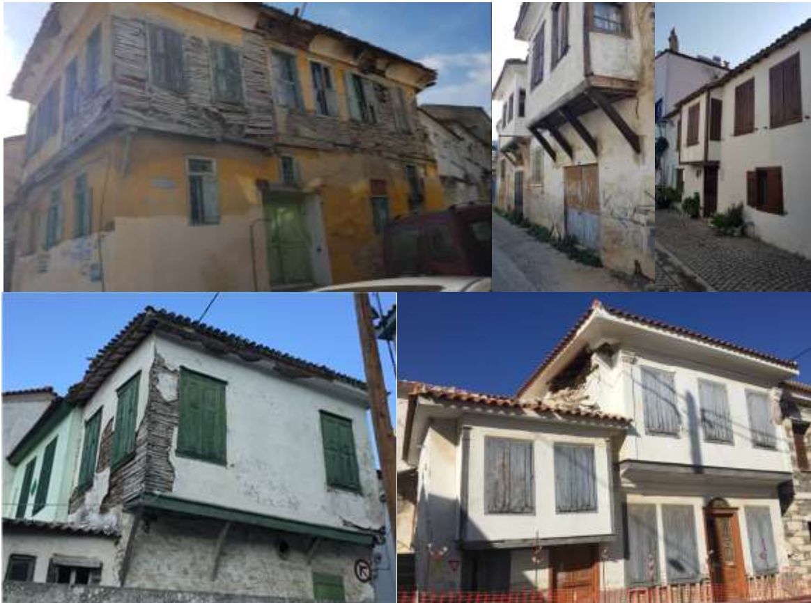
Figure 93: Some examples of hımsı structures in the affected areas (top row) in Turkey and (bottom row) in Samos
