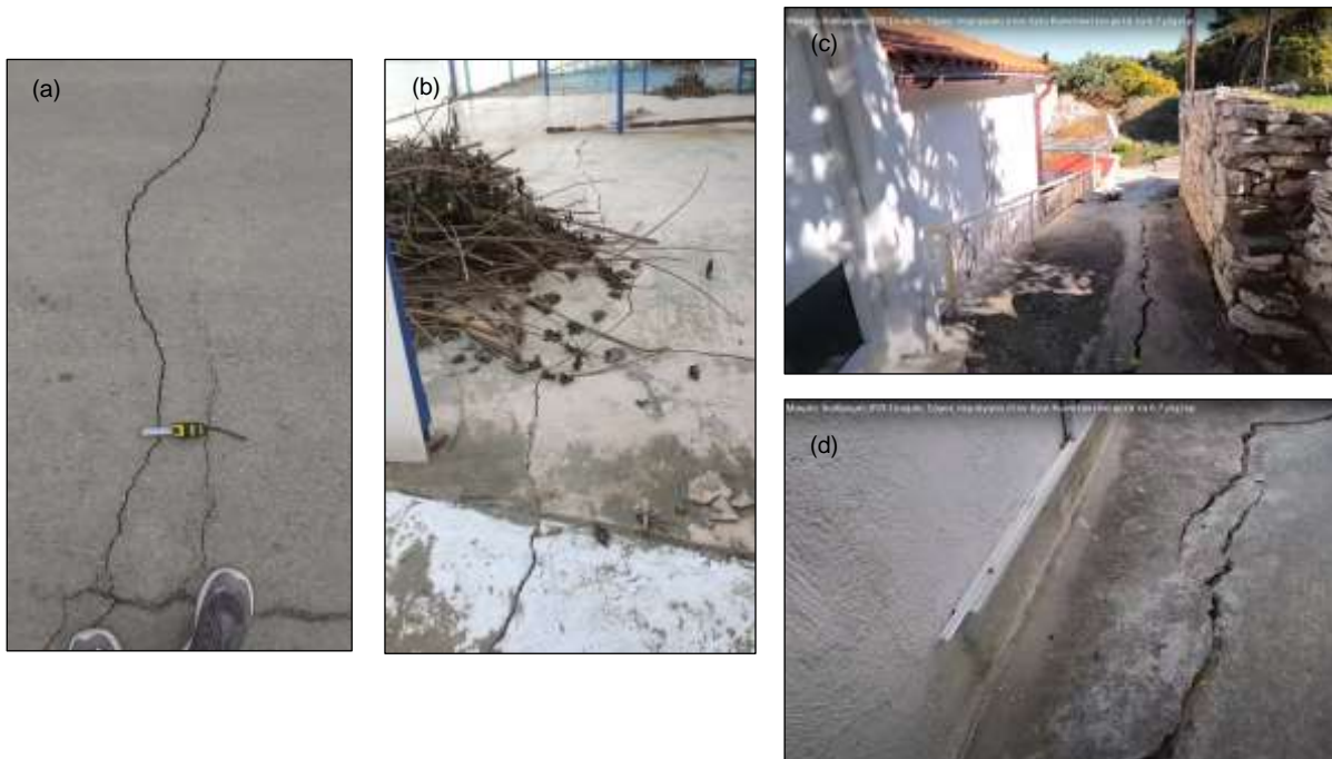
Figure 34: The observed ground cracks in a) Karlovasi, b) Kokkari and c) and d) at the village of Agios Konstantinos (source: https://www.youtube.com/watch?v=E5lv20MwagI&t=1s )
