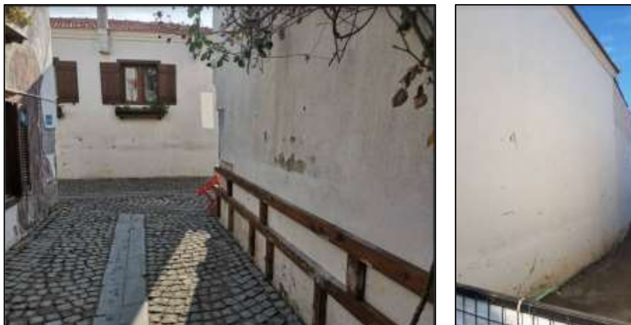
Figure 105: Buildings surveyed in Sığacık (coordinates: 38.1944937, 26.7854733).
