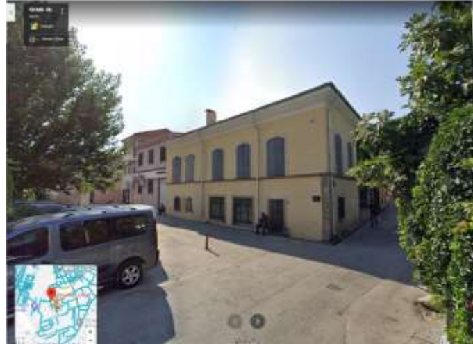
Figure 77: Street view from Izmir Two storey load bearing masonry buildings
