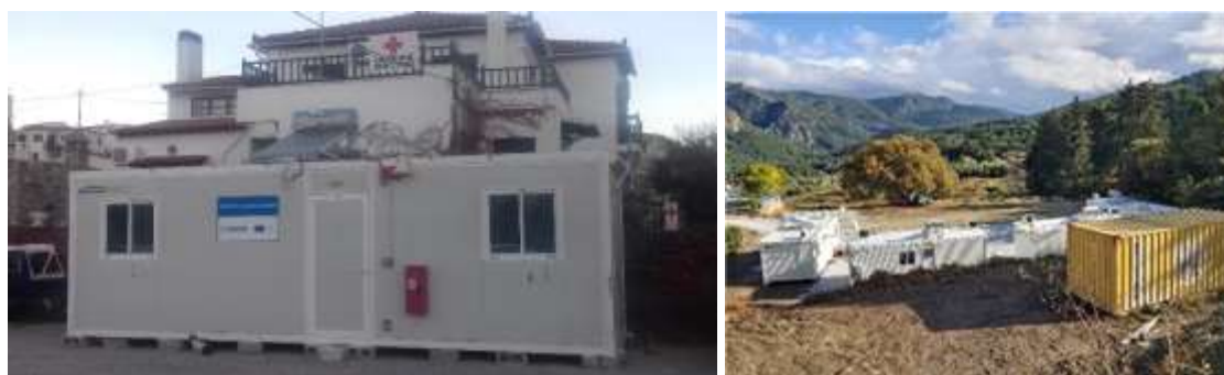
Figure 120: Container used as infirmary at Kokkari (samos2000goal, 2020); settlement of containers at Konteika
