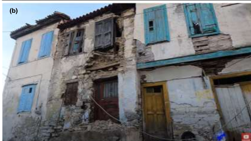
Figure 92: (a) Schematic representation of a timber frame (after Diri, 2010) and (b) two buildings with stone infill (the building in the middle) and bagdadi cladding (the building on the right) (from "Mikres diadromes" youtube channel)
