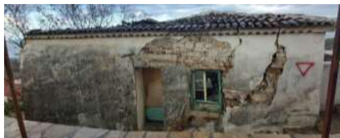
Figure 66: Diagonal shear cracks to the walls with different widths.
