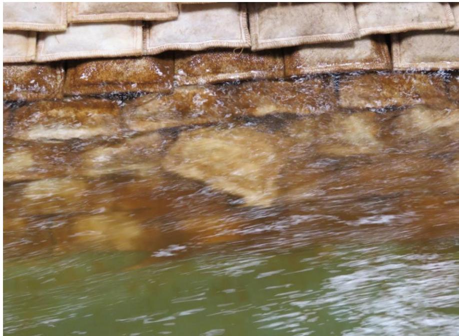
(b) Pull-out of a geobag from a layer close to water surface
