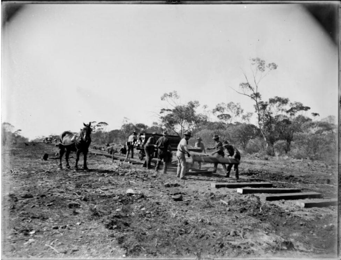
Figure 14: Railway construction in 1911. Laying sleepers over a formation that has required little preparation. To the rear of the wagon, men are securing temporary rail to the sleepers, while in the far distance a locomotive waits. Source: State Library of Western Australia 013933PD
