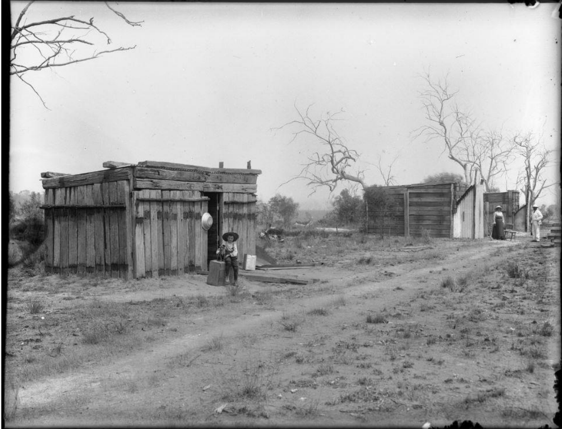
Figure 17: Gangers huts at Youraling, 5km north of Brookton. A gang would have been located here once construction had passed, probably around 1887. The use of local materials in the construction of the huts, such as railway sleepers, is typical. Workers camps provided opportunity for line maintenance and, though not this one at Youraling, occasionally grew into small towns. Source: State Library of Western Australia Call No.5323B/387
