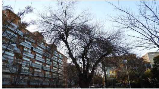
Built blocs in stages 1 to 3
