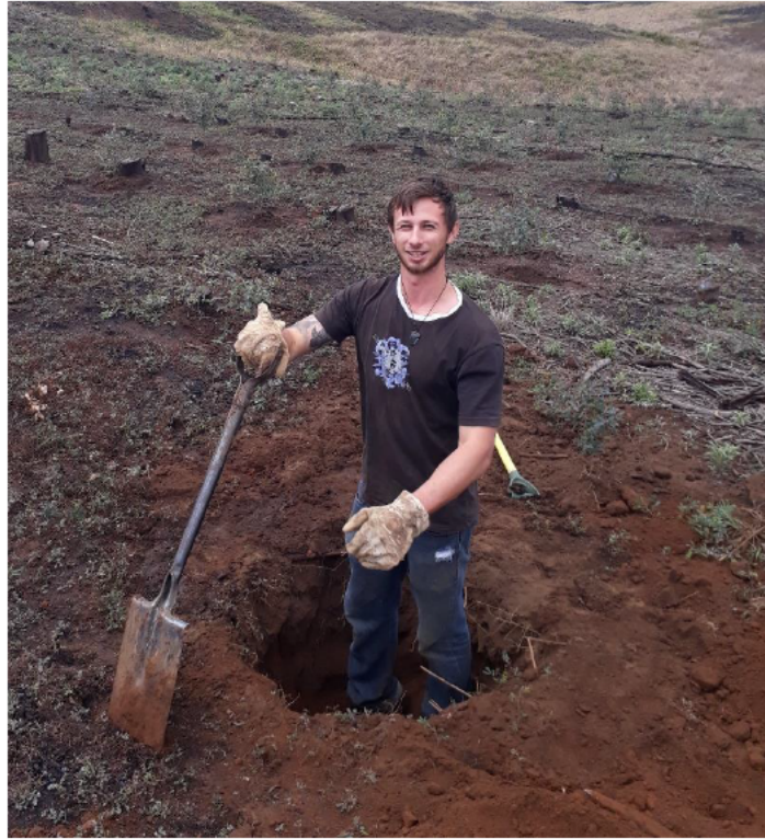
Plate 3.6: Storage tank hole being dug by Jordan Bull.
