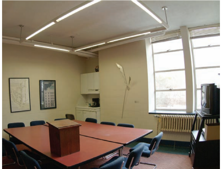
Bill 212 before renovation, Spring 2008
