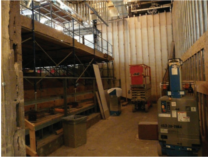
Bill 106 temporary construction floor and mechanical lift, as viewed from the front of the room, Summer 2008
