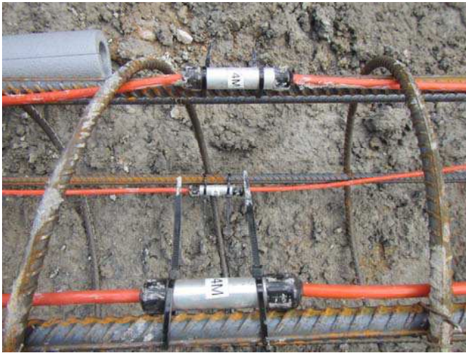
Figure 7. Detail of thermistor strings installed on the steel cage at 22 Station Road.
