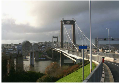
Fig. 3. The Tamar Bridge.
