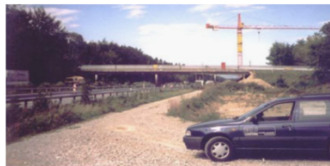
Fig. 9. View of Z24 Bridge.
