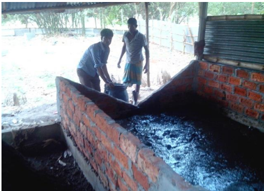
(a) Loading bio-drying units with pre-treated FS
