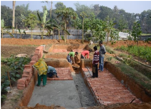
(a) Drying beds – masonry work
