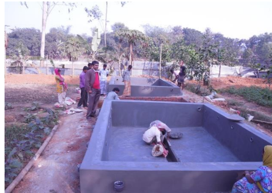
(b) Drying beds – plastering work
