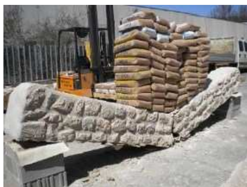
Figure 24 – Failure of a stone masonry ring beam
