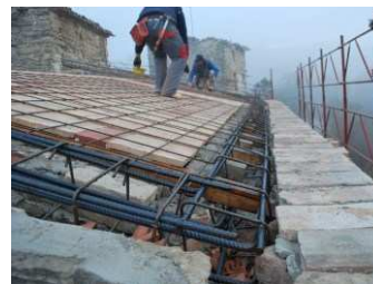
Figure 18 – Examples of reinforced concrete ring beams
