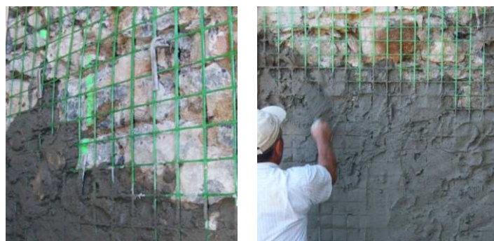
Figure 5 – Application of the mortar
