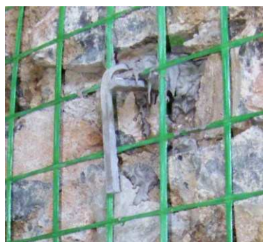
Figure 4 – Detail of the GFRP L-shaped bar
