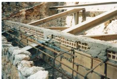
Figure 18 – Examples of reinforced concrete ring beams
