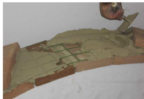
Figure 15 – Detail of reinforced arch
