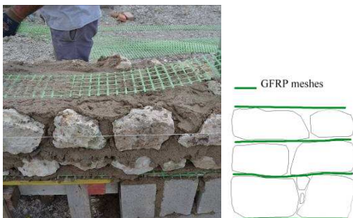
Figure 20 – Stone FRCM ring beam
