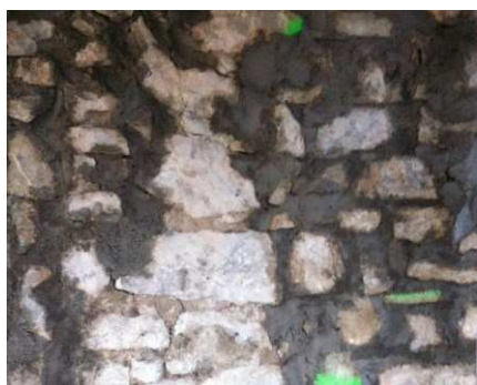
Figure 3 – Mortar joints repointed with new mortar
