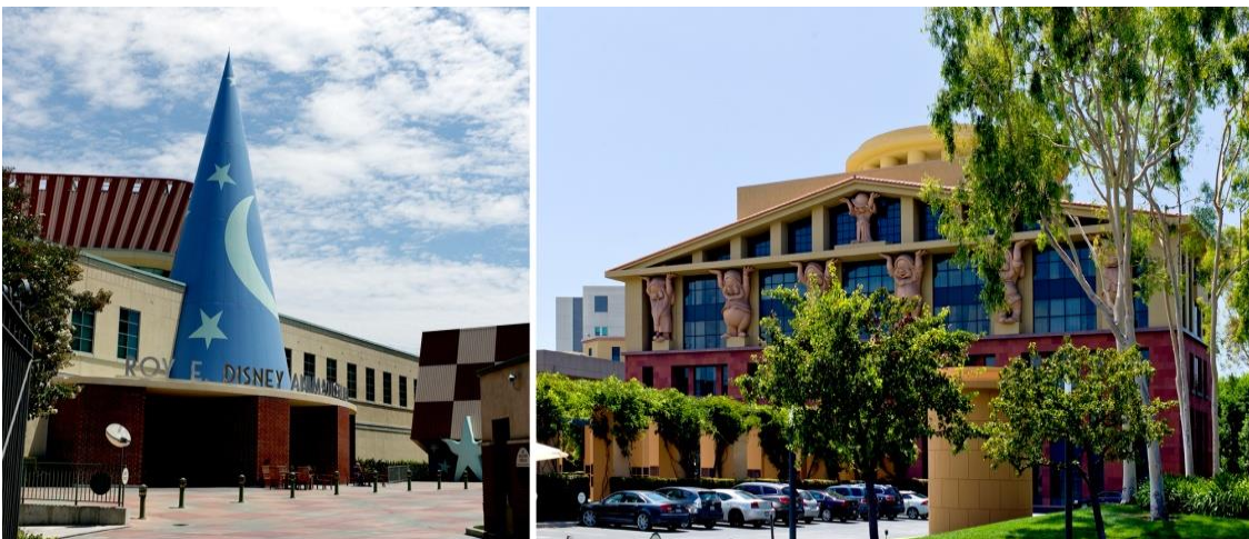
Figure 15. The Disney Feature Animation Building designed by Robert A. M. Stern, 1995; Michael D. Eisner Building designed by Michael Graves, 1990,
