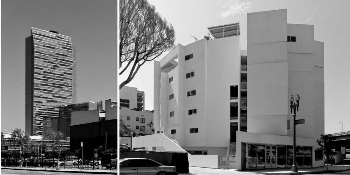
Figure 5. The high-rise designed by Gensler, 2010; New Carver Apartments designed by Michael Maltzan Architecture, 2009
