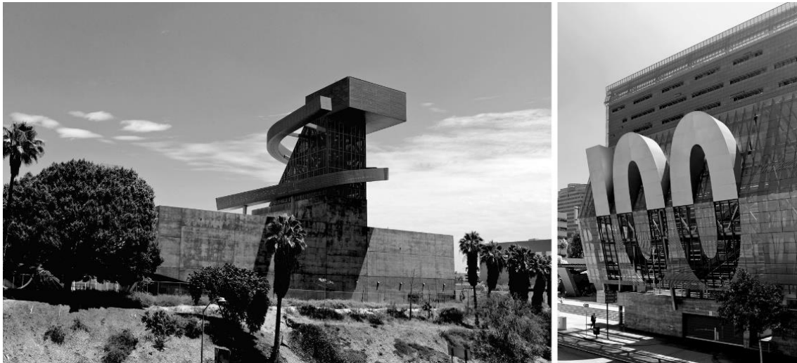
Figure 4. Central Los Angeles High School 9 for the Visual and Performing Arts, designed by CoopHimmelb[au], 2008; Caltrans District 7 designed by Thom Mayne, 2005
