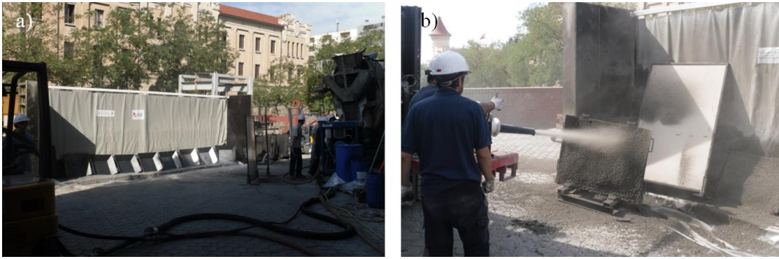
Fig.6 Special outdoor area to spray concrete: a) general view and b) detail of the spraying.
