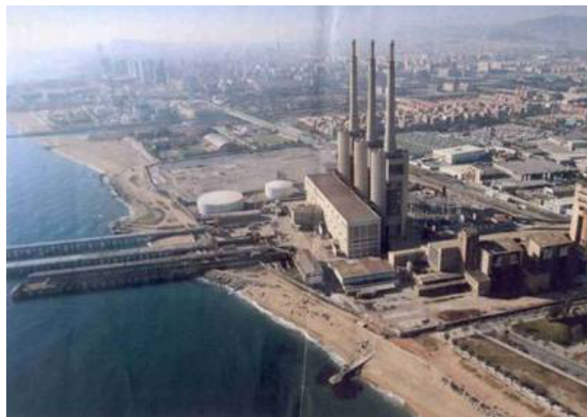
Figure 1 the existing Installation in 2004
