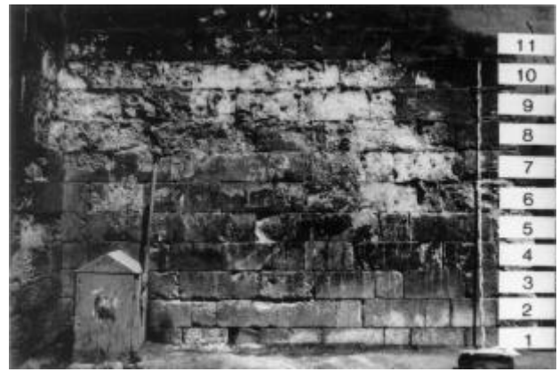
Figure 10. El-Merdani Mosque – Cairo/Egypt. Lower part of the SE-facade with numbering of rows of dimension stones.
