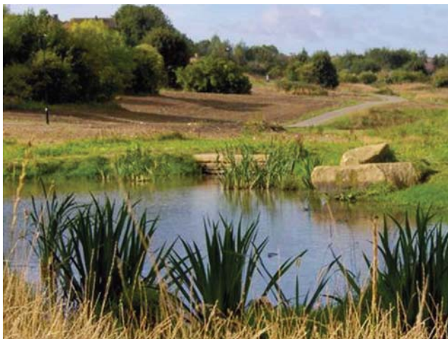
Figure 9. Example of a wet detention pond (CCC, 2009)
