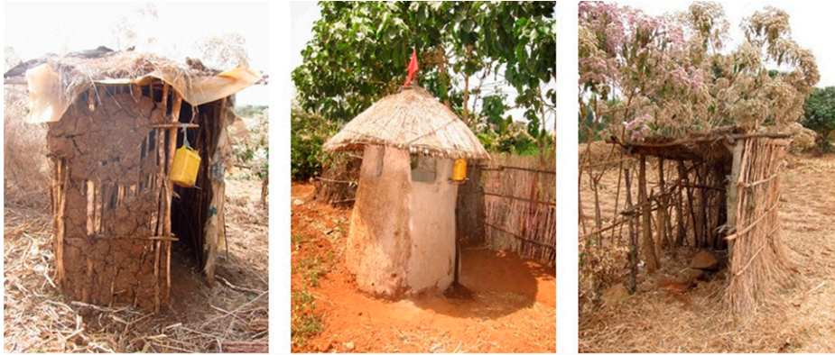
FIGURE 1. Examples of household pit latrines built in rural areas of Amhara Region, Ethiopia (Photo credit: William Oswald).
