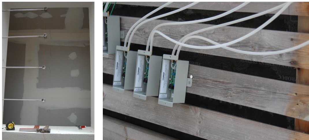
Figure 6-12. Positioning of the bidirectional probes at the centreline of the window (left) and their connection with the differential pressure transducers placed in the west compartment wall (right).
