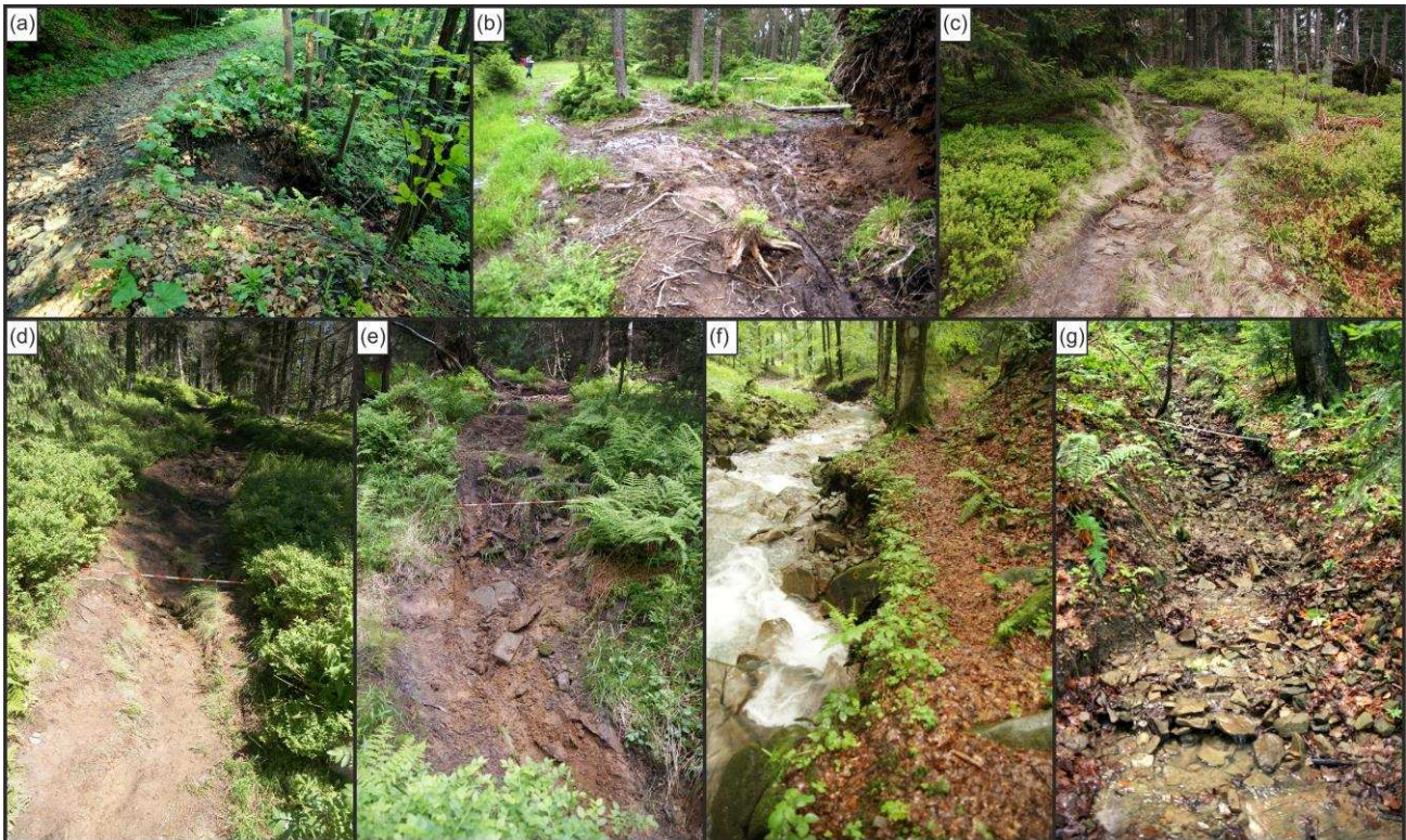
Figure 2. Examples of impacts in Gorce National Park related to the extreme rainfall event in May 2010: (a) damage to trail tread due to small landslide; (b) creation of muddy sections; (c), (d), (e) development of erosional rills destroying trail tread; (f) undercutting of trail treads by a stream; (g) increase in delivery of sediments due to soil erosion.
