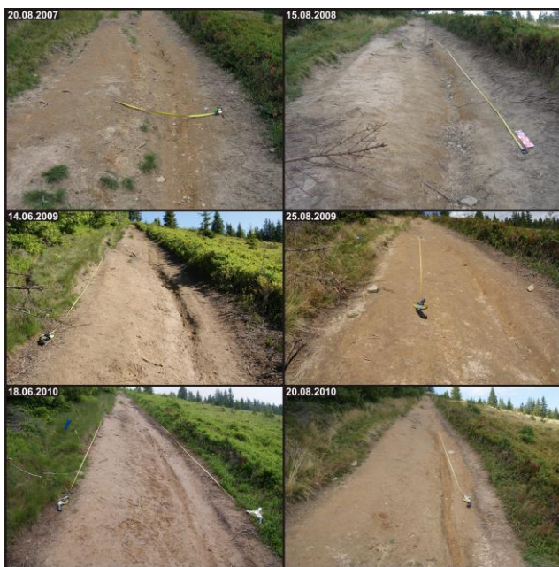
Figure 6. Case study E – an example of trail which had already been degraded before the intense rainfall event. Trail tread was uneven and wide. The extreme rainfall event caused an increase in soil erosion and the rill was deepened.
