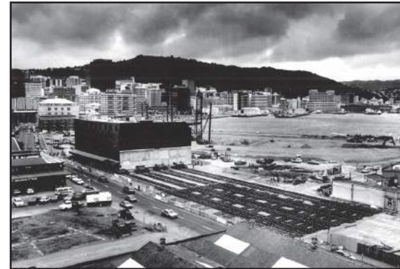
Fig. 8.5: 1993 - Museum Hotel moving 120 meters to clear the site for Te Papa Tongarewa to begin construction.
