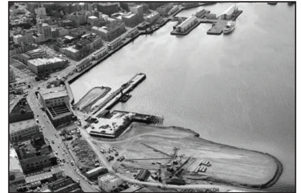
Fig. 8.2: 1968 - Land reclamation for the Trans-Tasman roll-on roll-off terminal. Te Papa's site to be.
