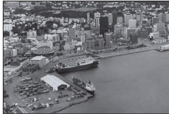
Fig. 8.4: 1969 - Completed Trans-Tasman Terminal and shed 26
