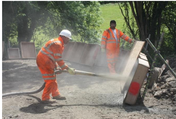
Figure 2 Spray operations at contractor's yard
