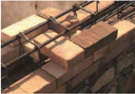
Figure 3. Example of a brickwork steel-reinforced ring-beam.
