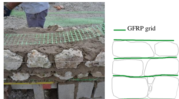
Figure 10. Construction of stone ring-beam strengthened with GFRP grids.
