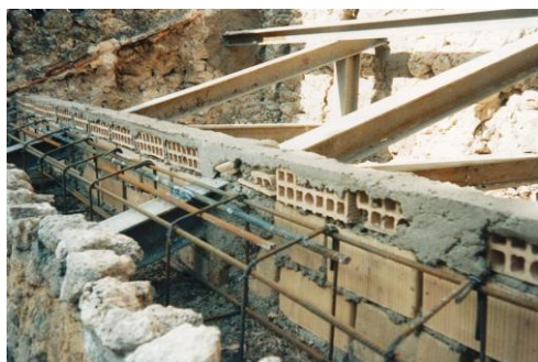
Figure 1. Example of a RC ring-beam.
