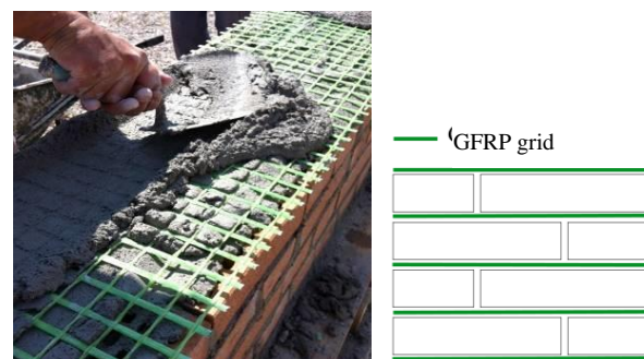
Figure 11. Construction of brickwork ring-beam using a GFRP grid.
