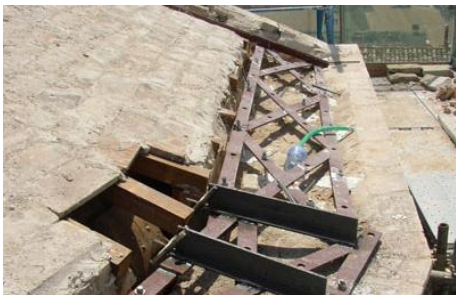
Figure 4. Example of a steel-profile ring-beam.
