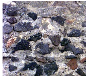
Figure 16. Tuff masonry arrangement of the goat house of the Royal Palace of Capodimonte.
