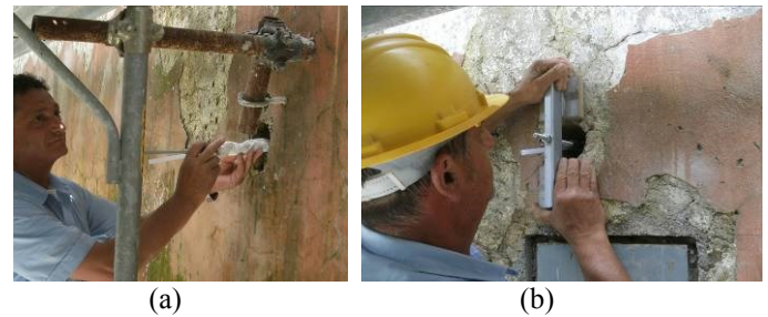
Figure 20. (a) Insertion of the steel bar; (b) pre-load application.
