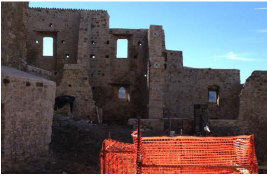
Figure 11. Main entrance of the castle where the connectors have been applied.
