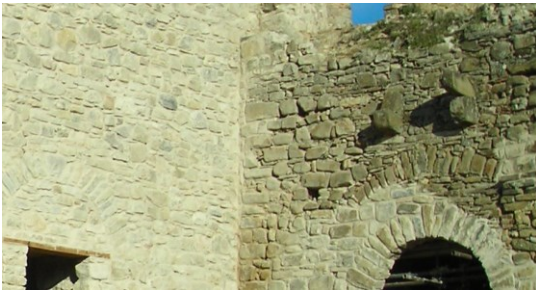
Figure 12. Masonry arrangement of the Laurenzana castle.
