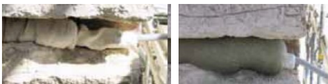
Figure 4. Different phases of the grout injection of the fabric bag-case.
