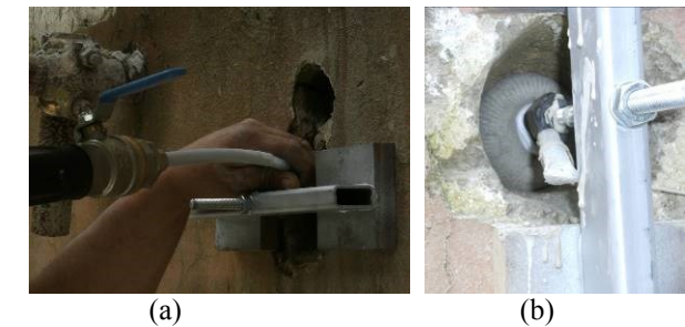
Figure 21. (a) Grouting operation; (b) the reinforcement during curing time.
