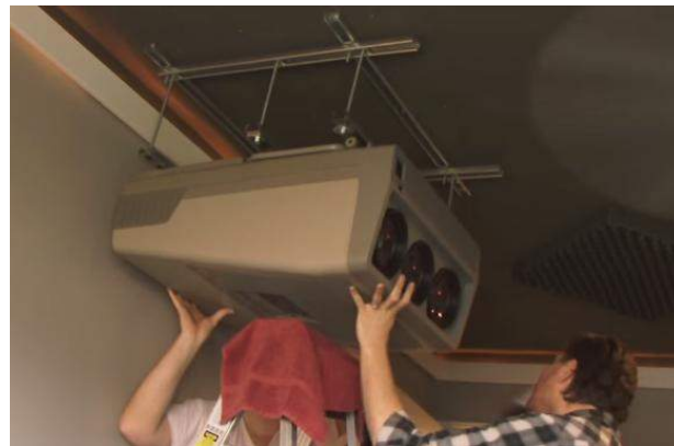
Figure 88: a CRT projector during installation (Kennis Russell, 2014)
