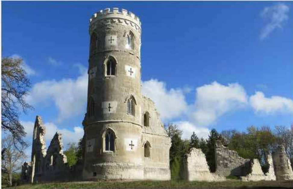
Wimpole Gothic Tower, after conservation of all masonry and replacement of crenellations and arrow slits
