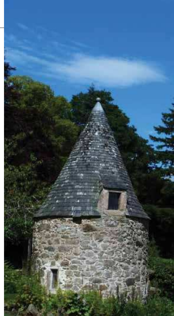
▲ Replacing cement render with replica feebly hydraulic hot-mix lime harling and lime wash at 17th-century Craigievar Castle, Alford, Aberdeenshire
