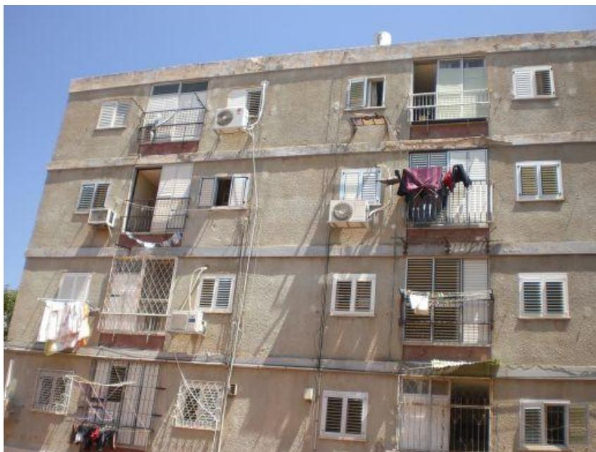
15. Neighbourhood Renewal Project before. This is how the building in 132 Weitzman Street in Raanana looked before major renovation. The renovation includes strengthening of its foundations against earthquake, the creation of larger apartments, the addition of three storeys, with each current flat receiving an additional room and balcony, and for the whole building an elevator and a lobby. Source: Liran Sahar, 10 July 2011 <http://www1.bizportal.co.il/article/277784>.
