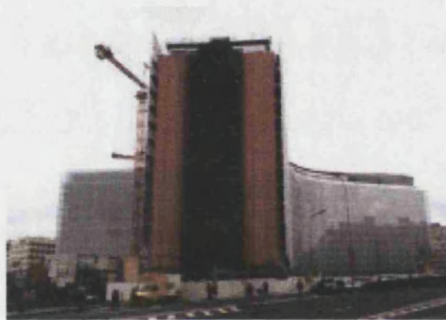
Renovating the Berlaymont
