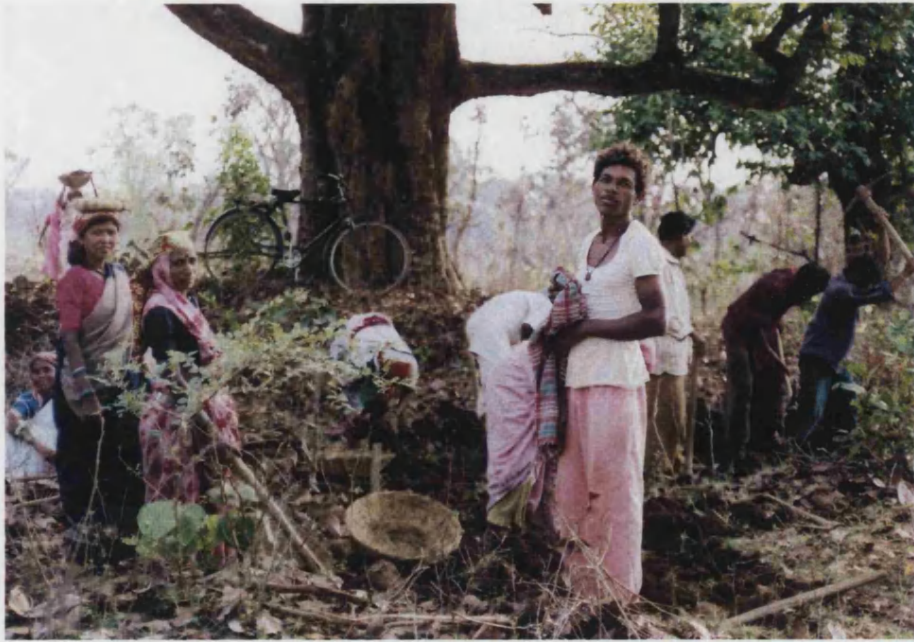
Plate 19: Markakasa people digging earth to build a road.
