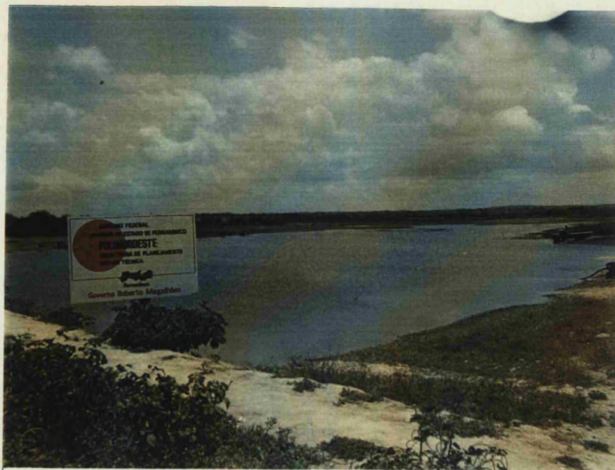
Plate 3. A small Dam constructed with POLONORDESTE resources in the Northern Agreste
