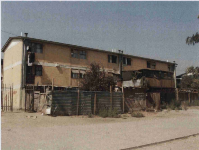
Photo -2. Housing Extension in Santa Teresa
