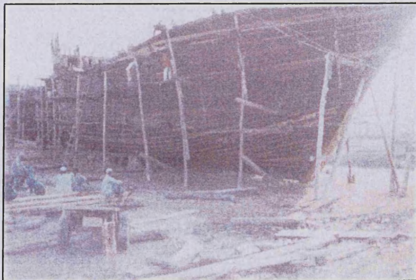
Plate 15. Scaffolding around a hull.
