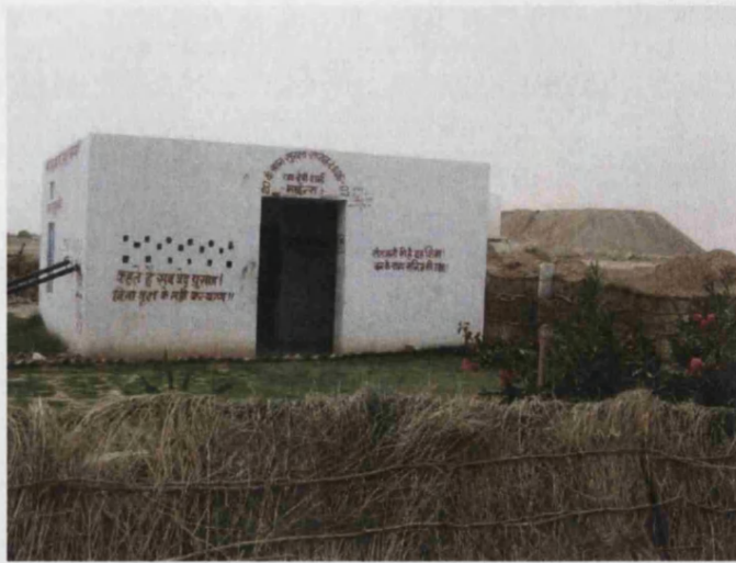
Plate 8. The Rama Devi Sharma mine office.
