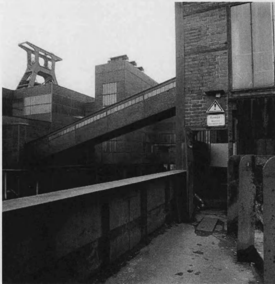
Fig. 9.4: Shaft XII – Coal Wash and Hoist Frame 3
