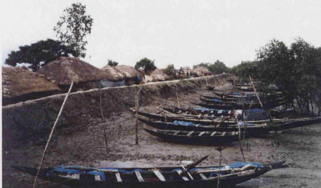
Huts and boats separated by bund. During high tide, river water reaches dangerously near the top of the bund.
