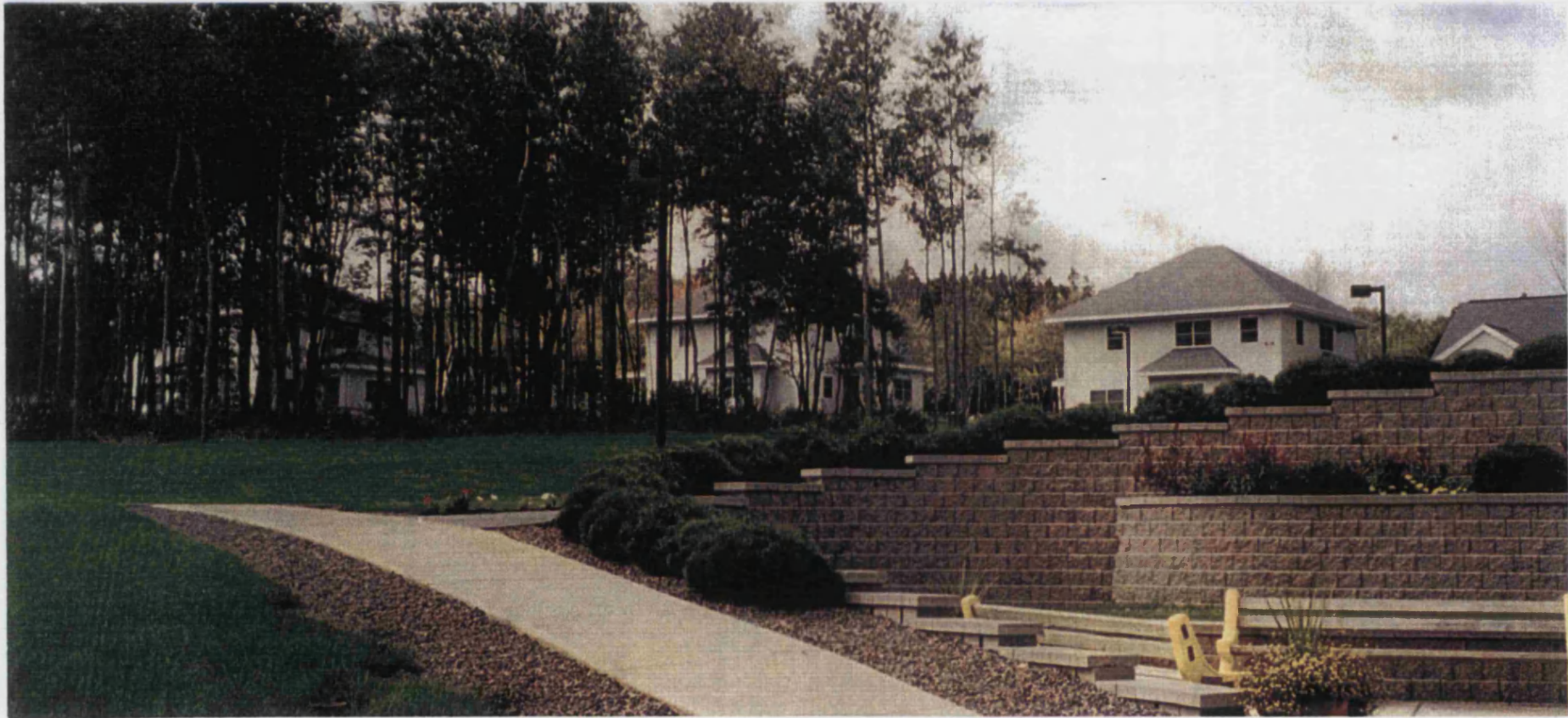
Nova Institution for Women, Nova Scotia. Part of the living accommodation, seen from the administration building. photo: S. Hayman
