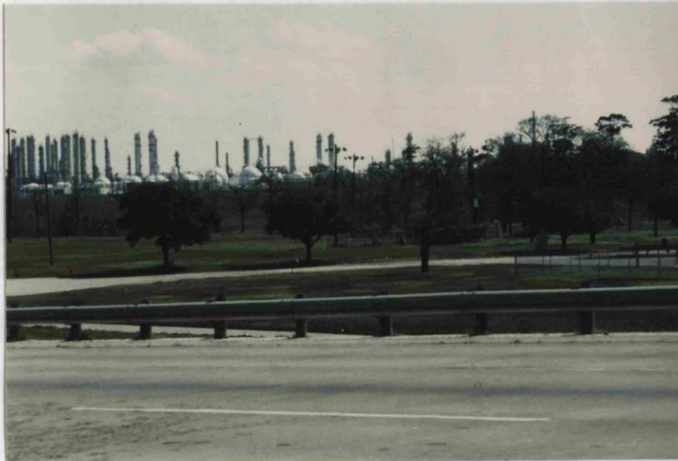
Plate 4.6 What could be a 'pure' pastoral scene in the San Jacinto Monument Park is abruptly disrupted by the presence of a solid background body of chemical establishments. Oil and gas processing plants are located within easy reach from main roads and the landscape these create has become typical of the east side of the city.
