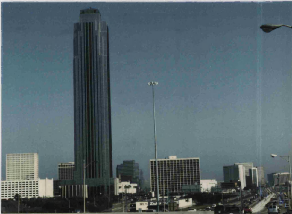
Plate 4.3 The Transco Tower, situated in a popular commercial sector of the city (the Galleria) is the site of oil-related offices and the tallest building in Houston. Looking like a chocolate bar, as it is popularly known, it is simply an eye-sore to the landscape. Impressive height and ostentatious presence of the Transco Tower epitomizes the embodiment of capitalist growth, flourishing business and powerful multinationals in the city.
