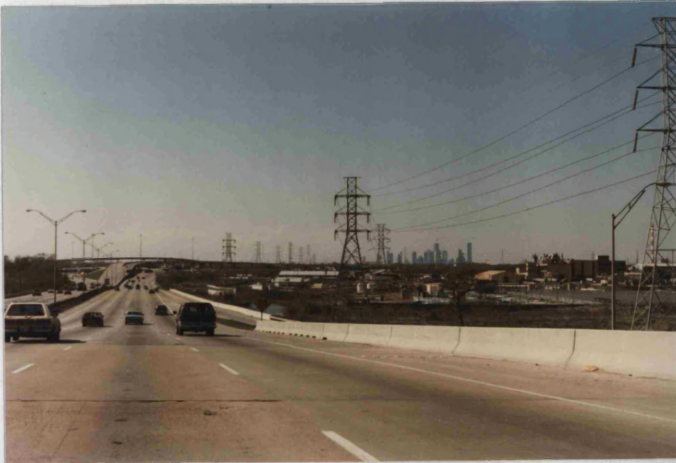
Plate 4.2 Typical Houston landscape, seen from the 610 Loop (see Figures 3.2 and 4.5) showing Downtown's prominent sky-line which contrasts the flat surroundings. After a pronounced turn on the I-59 high-way, the conglomeration of buildings in Downtown makes its sudden appearance like a cohesive, immobile monstrosity made of different shapes, heights, materials and colours.
