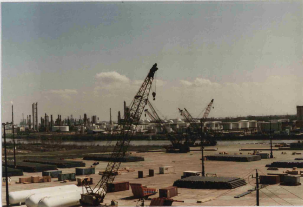
Plate 4.1 A view of the Ship Channel and the port of Houston displays the dominant presence of petrochemicals along the channel.
