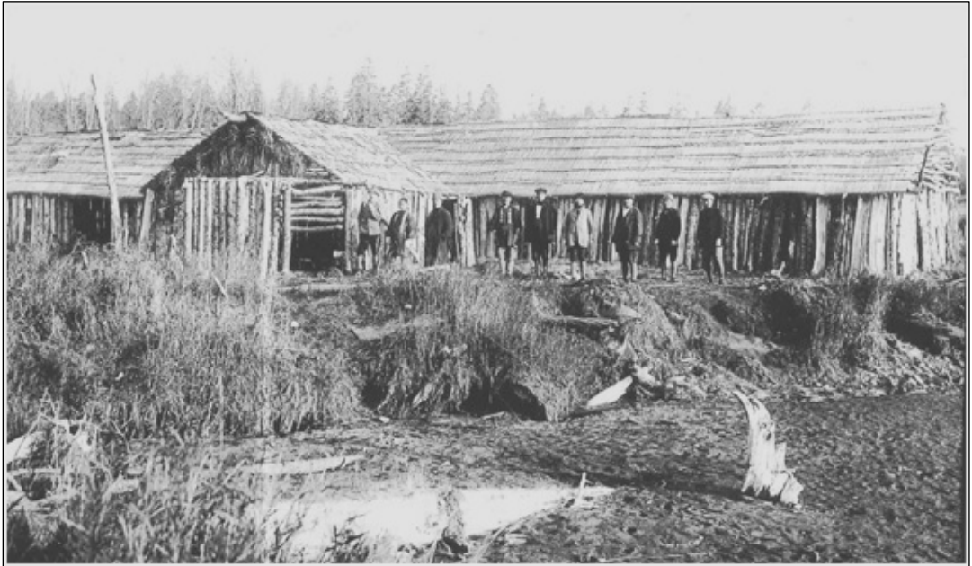
Image 6.3 – Temporary worker lodge ( hanba ) in Karafuto during a road construction project commissioned by the military in early 1920s
