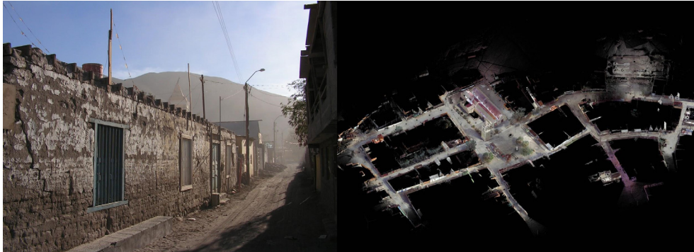
Figure 1: San Lorenzo de Tarapacá-Chile damaged after the 2005 earthquake (left) and after governmental reconstruction from the terrestrial 3D-laser-scanning obtained on-site in 2013 (right). (Source: Bernadette Devilat.)
