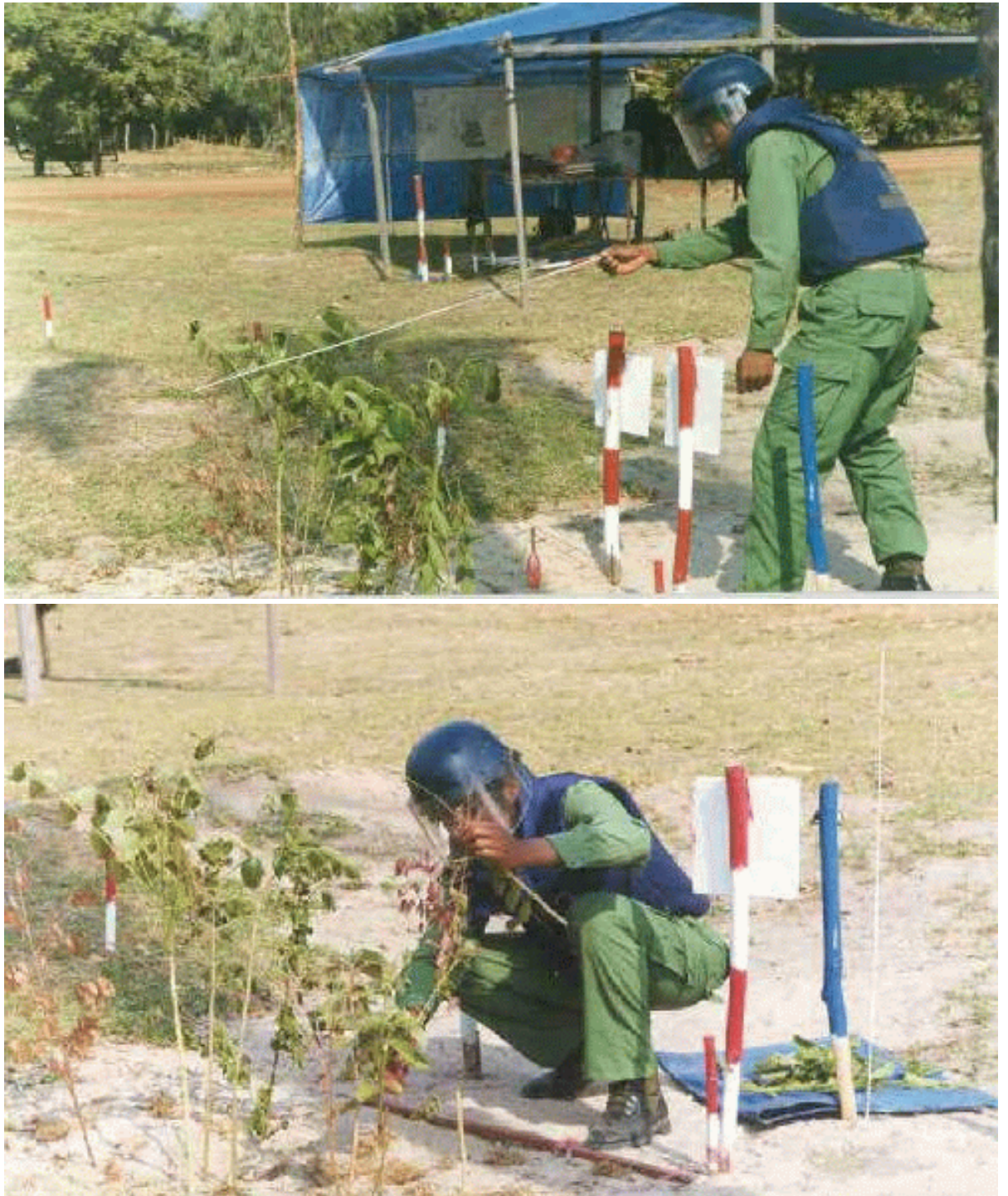
Figure 2.5: Sequence of operations, manual demining in Cambodia (part 1). — deminers demonstrating SOPs in a prepared safe area.
