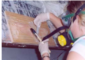
(k) Filling the larger changes in surface height with fibreglass strips
