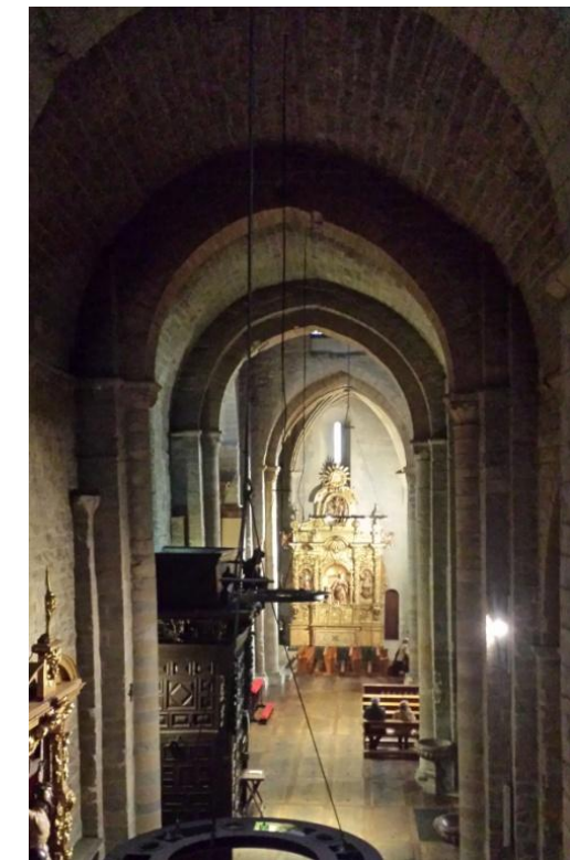
Img.40-41. Barrel vaults (the Epístola on the left and the Evangelio on the right.)
