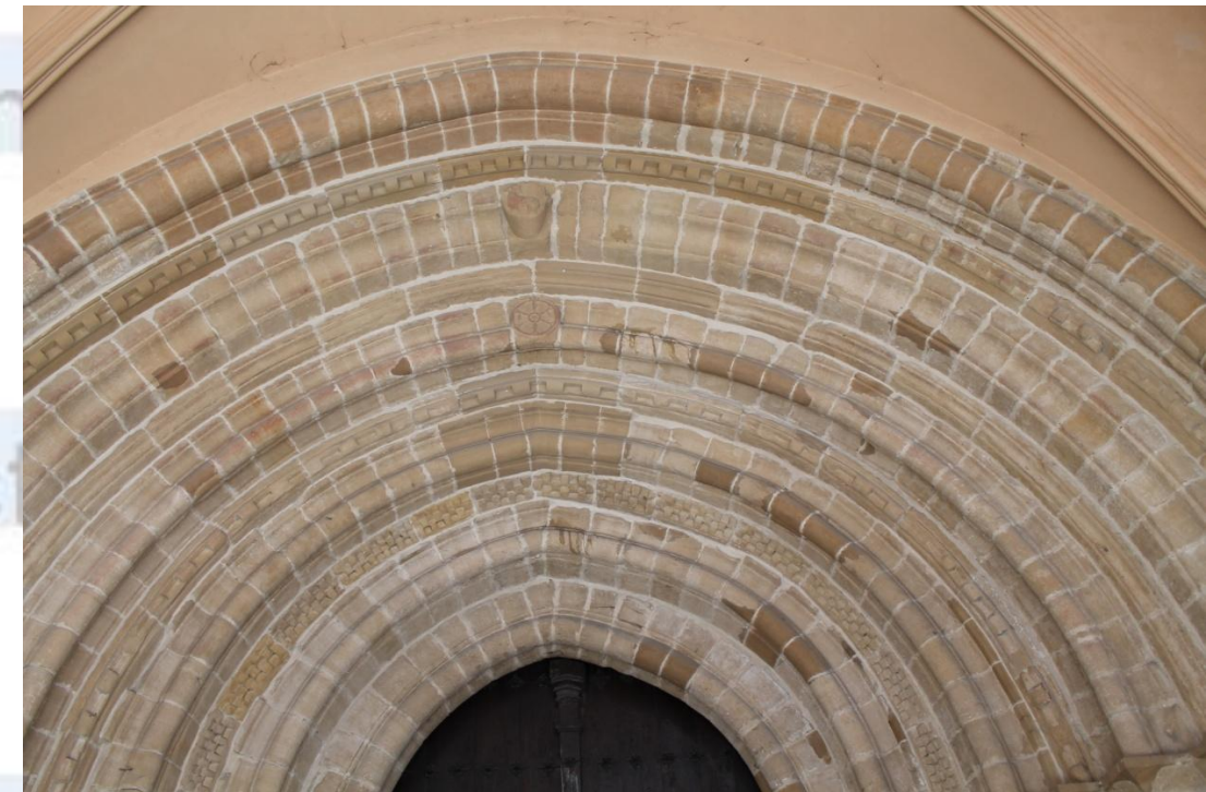
Img.61-62-63. Saint Miguel entrance
