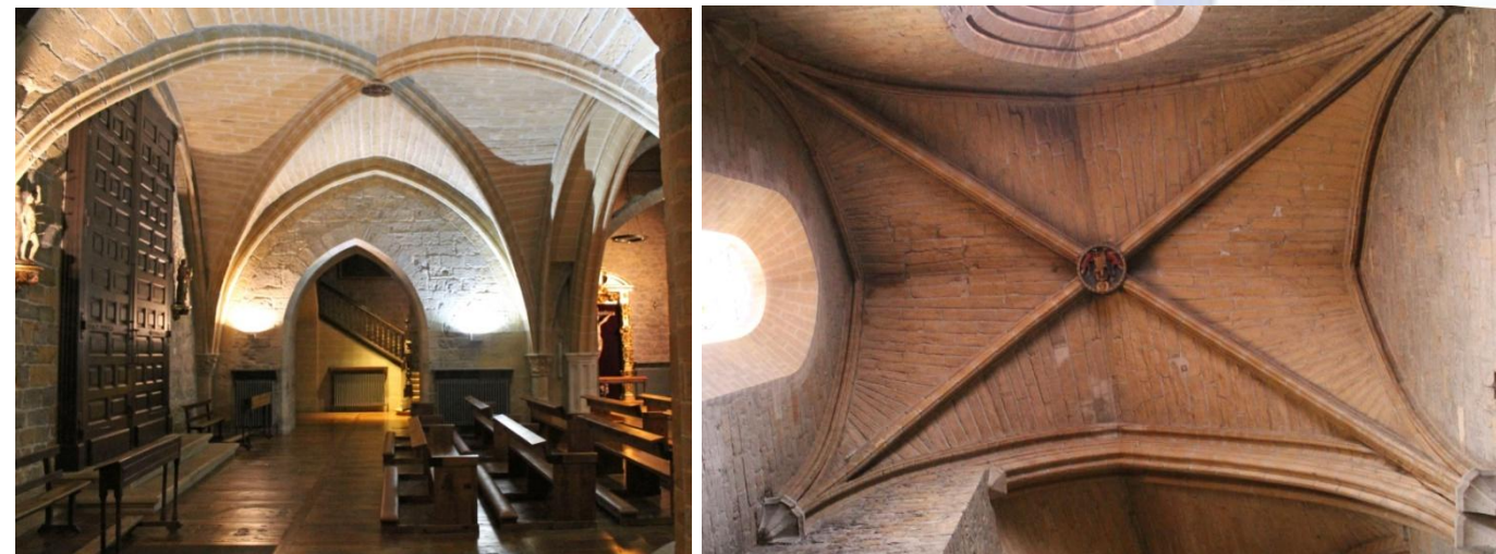
Img.36-37-38-39. ribbed vaults (the main nave and under choir on the left, the altar and Saint Miguel chapel on the right)
