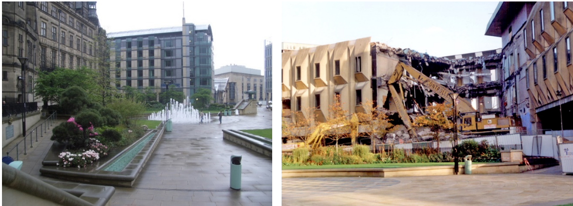
Figure 20: Sheffield Town Hall during the demolition of the old extension in 2002, and in 2010 with the Mercure St Paul Hotel
